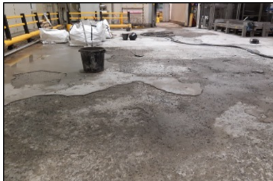
Surface preparation before ARC EG-1 is applied.
