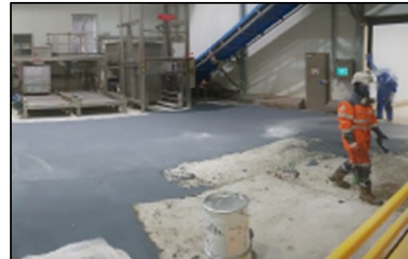
Floor after ARC EG-1 coating is installed.
